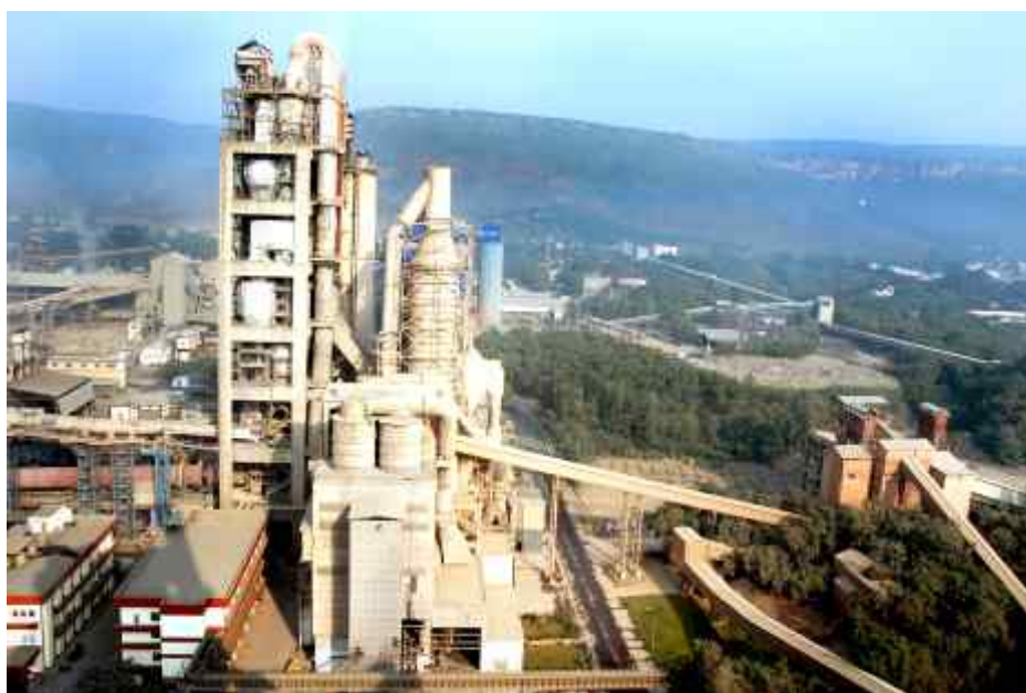
ACC Plant at Kymore, Madhya Pradesh, India where a joint project has been initiated by ICPE and ACC for co-processing of Plastic Wastes in Cement Kiln.
